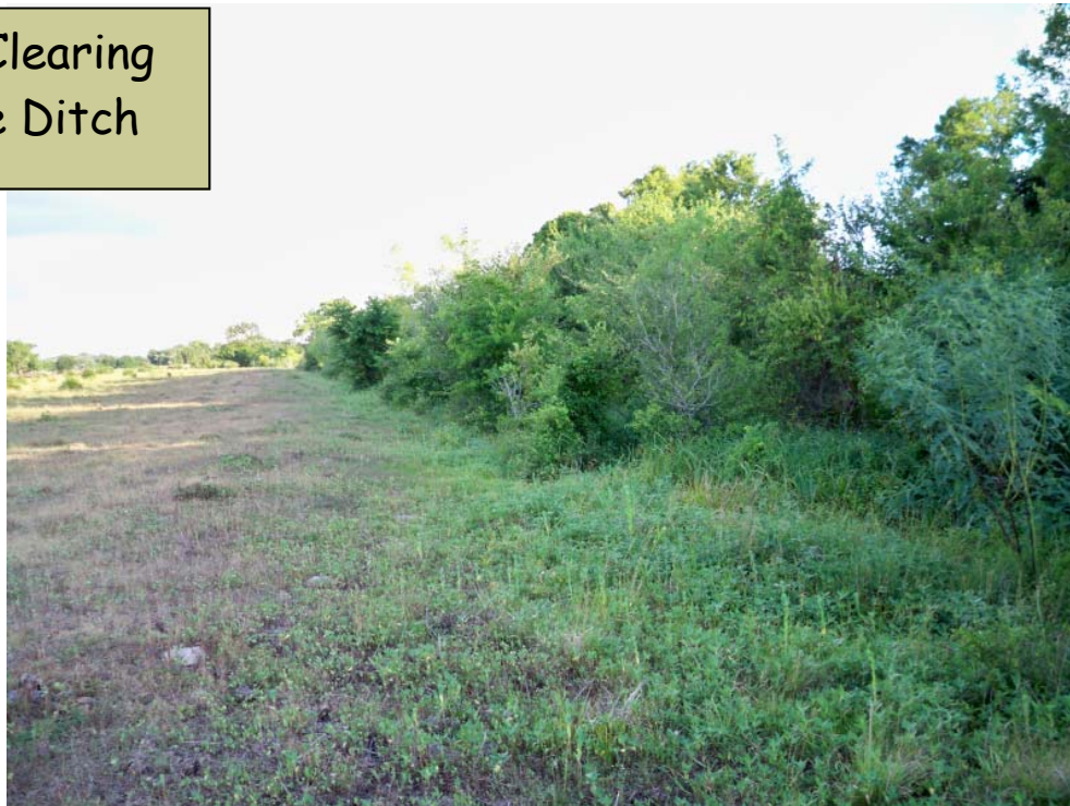
After Clearing Drainage Ditch
